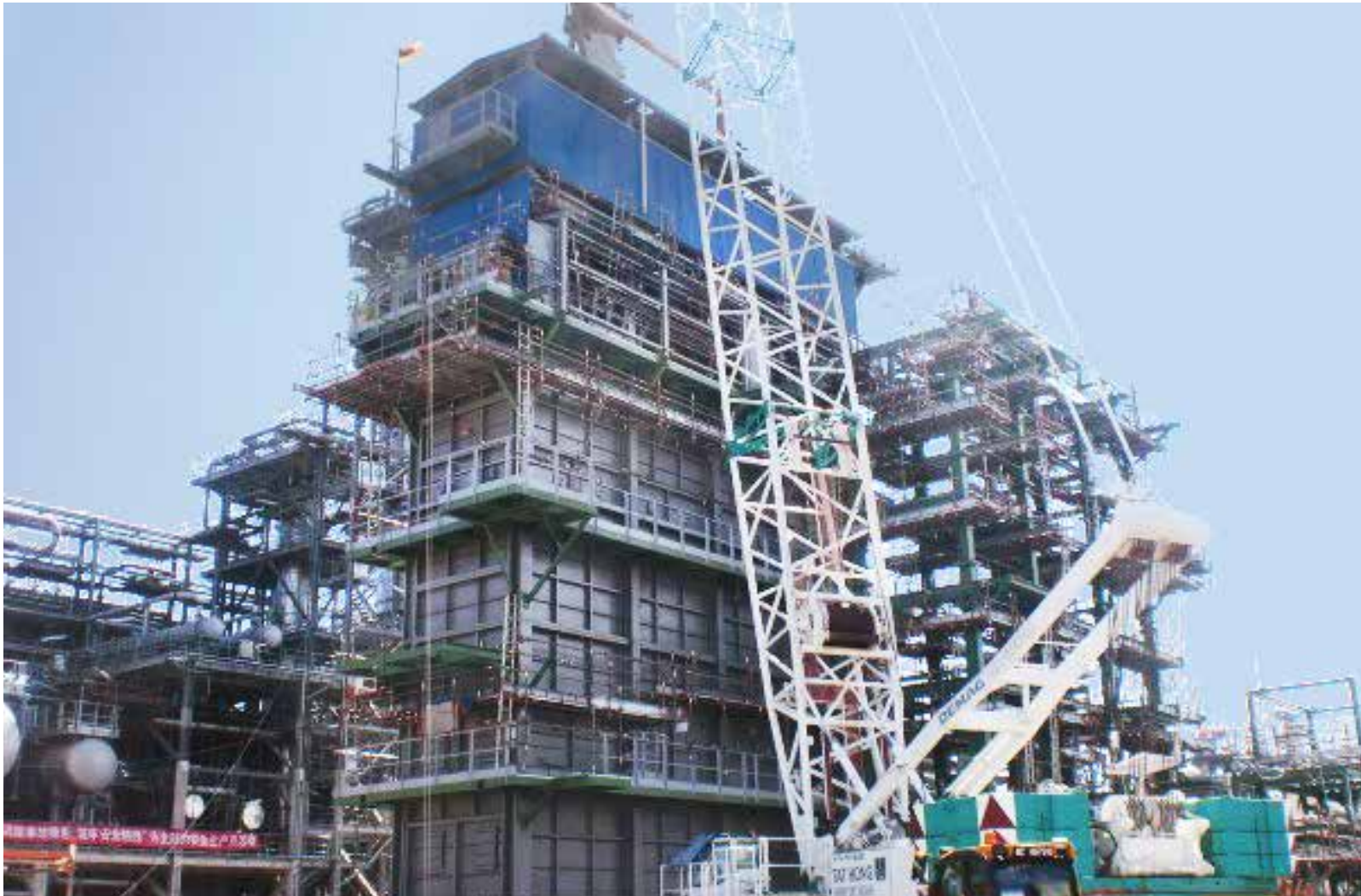
Supply & Fabrication of Hydrogen Manufacturing Unit (Reformer & WHRU) Hengyuan Refining, Port Dickson, Malaysia
