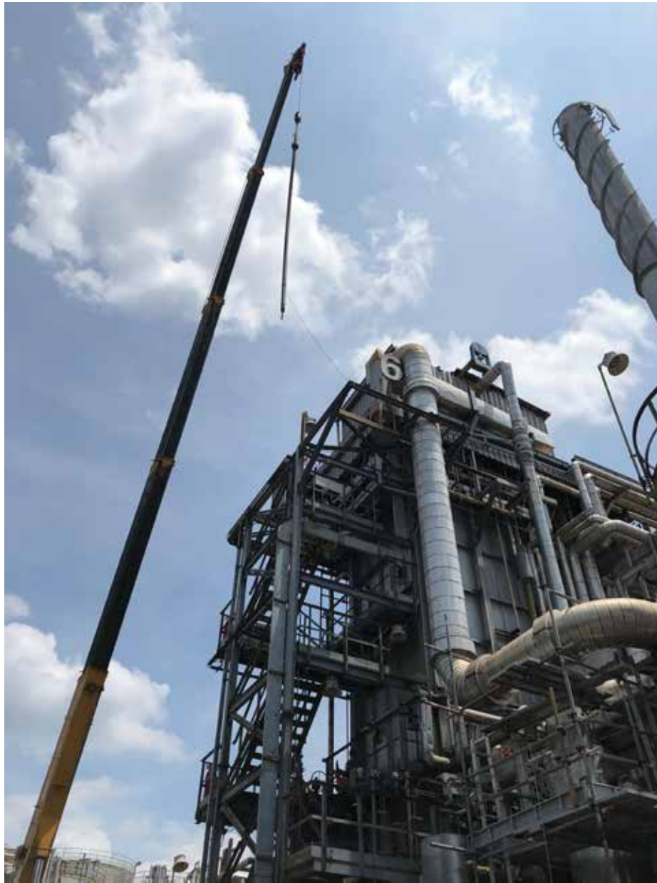
Replacement of Reformer's Tubes, Air Products Banting, Malaysia
