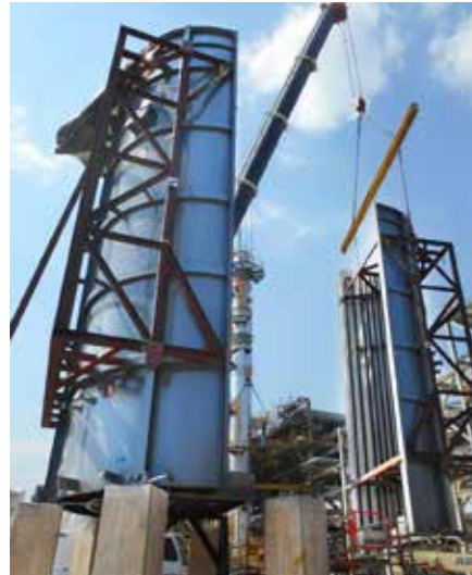
Fabrication Hot Oil Heater Package, ISMOCOL S. A. Colombia
