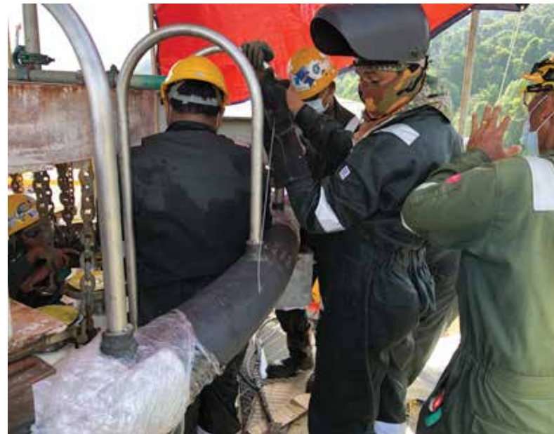
Replacement of Reformer's Tubes, Air Products Kuantan, Malaysia
